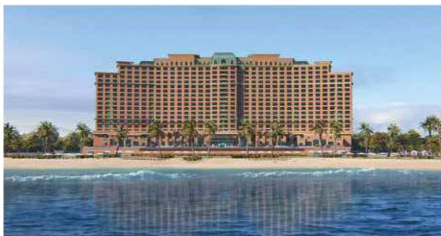
Greener Water Hotel project Negombo - under construction
